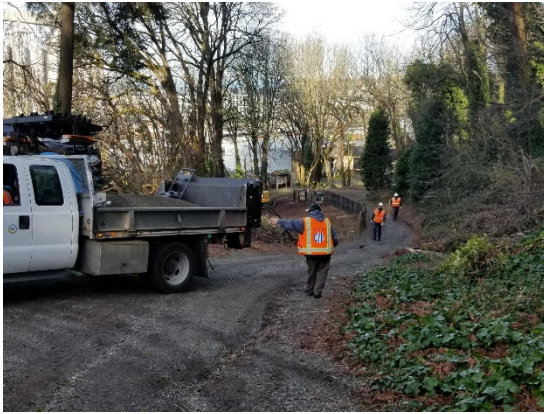
SDOT repairing gravel service road by filling in washed out sections
